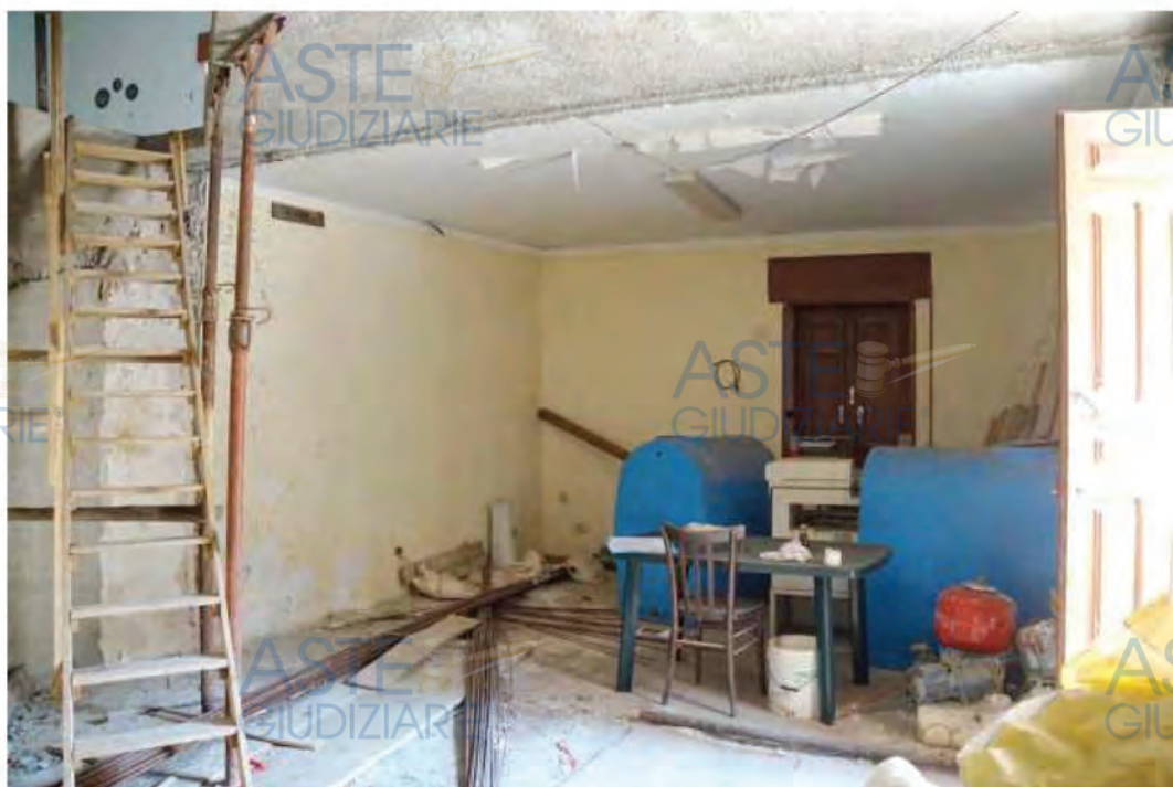
interno piano T
