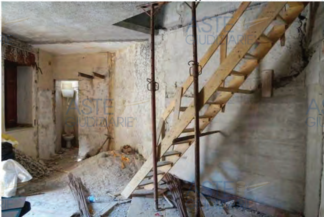
interno piano T
