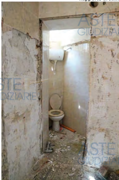
interno piano T
