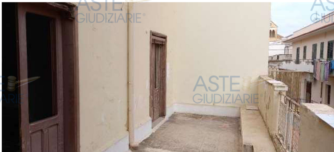
Foto 11 – Immobile “1A” – Balcone a I P
