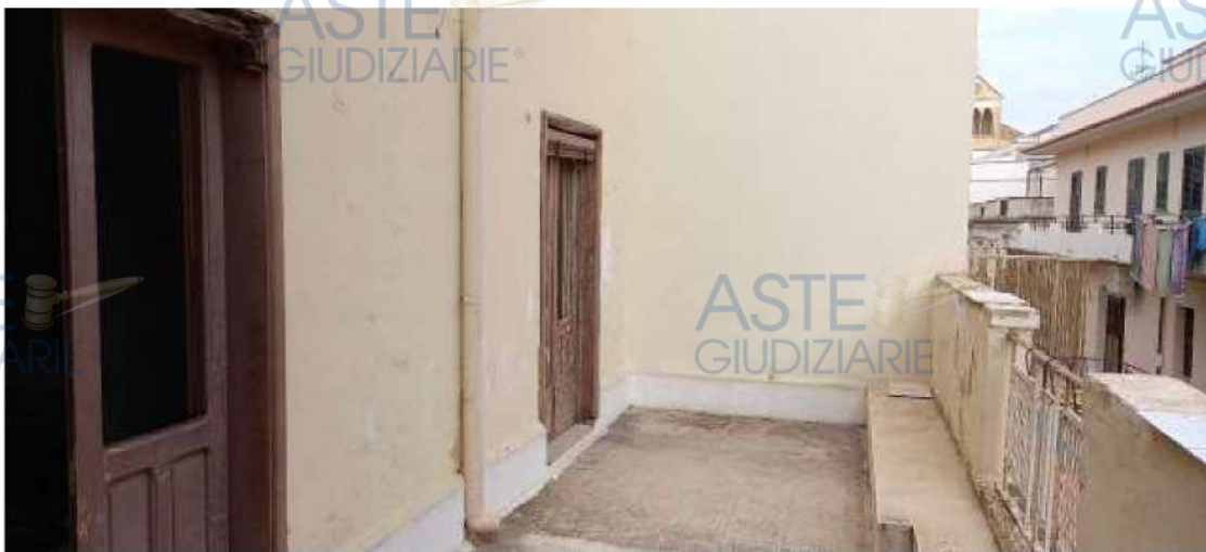
Foto 11 – Immobile “1A” – Balcone a I P
