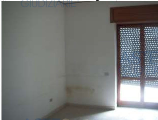
(foto 4: Vista camera)
