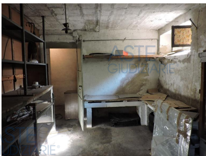
Cantina piano S1
