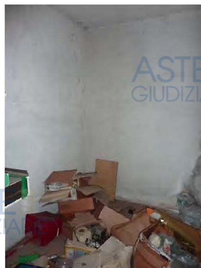
Locale cantina sub 5 piano interrato
