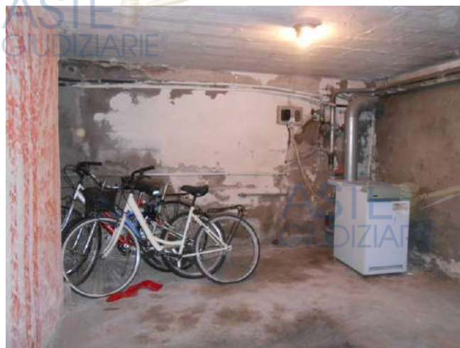
Piano Interrato c. termica
