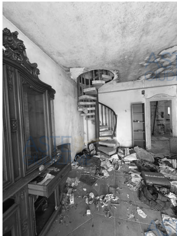
Salotto al piano terra (villa p.lla 256, sub. 1)
