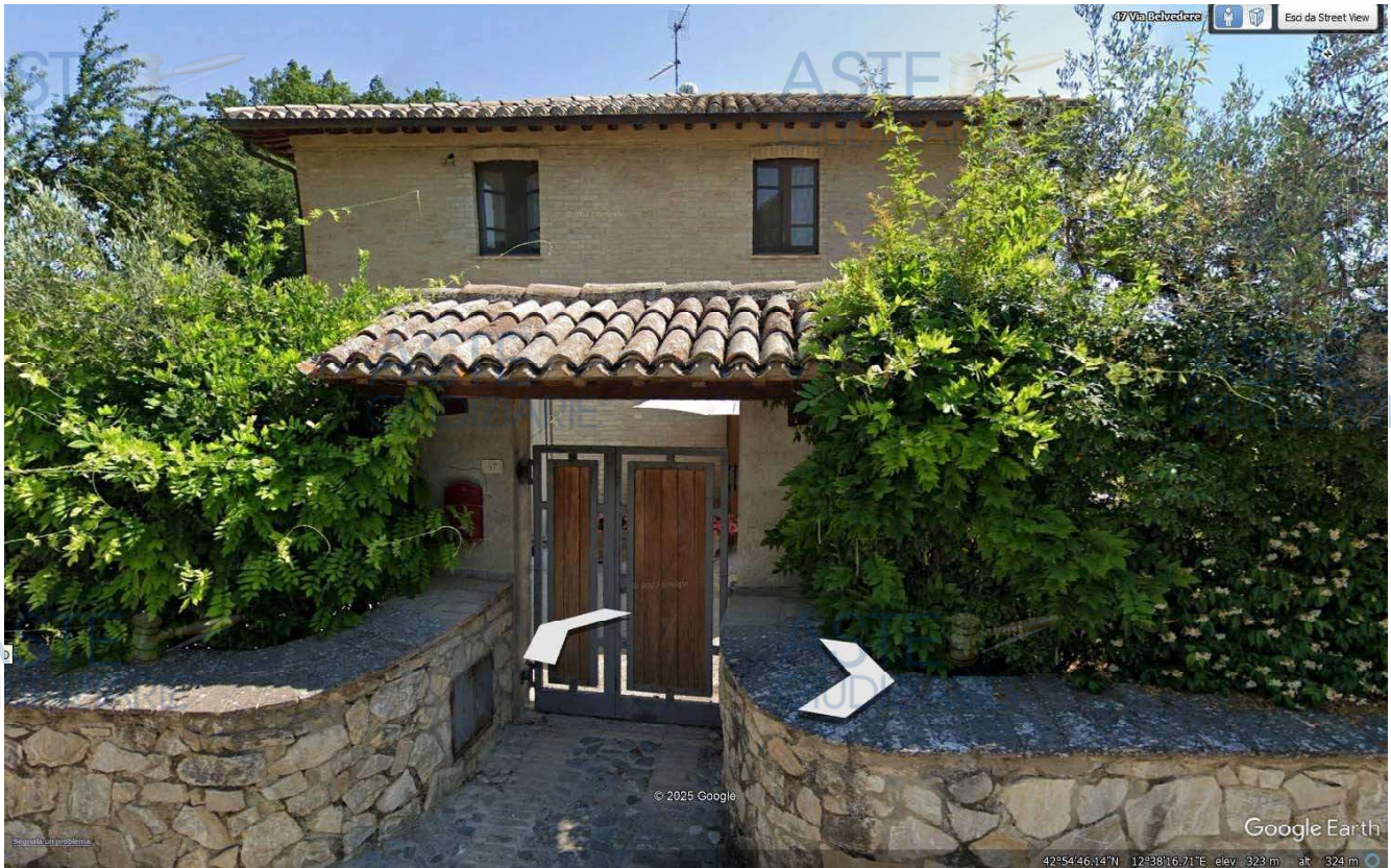
Vista da google street view
