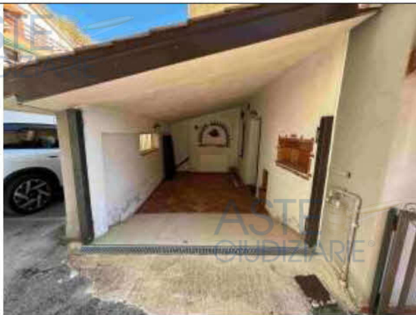
Piano terra- Vista box auto
