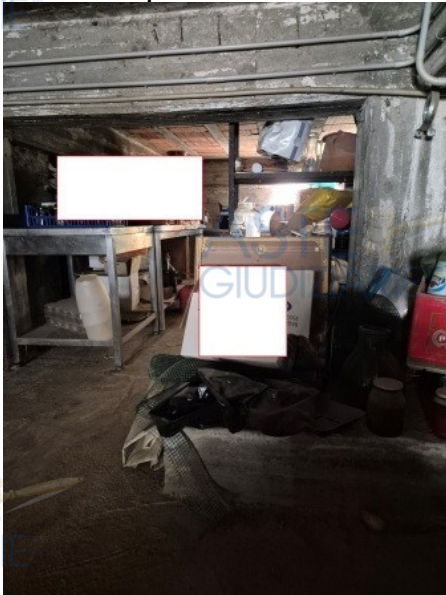
Figura 34 cantinola 1 piano seminterrato
