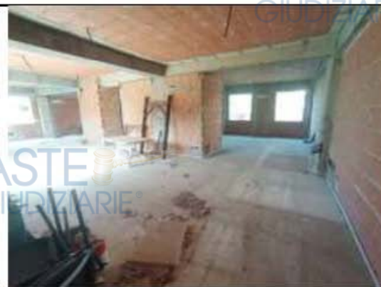
Piano seminterrato interno N-E
