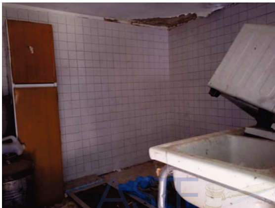
Part. 405 sub 5 - Vista interna piano seminterrato
