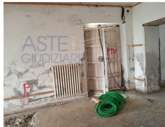
Part. 504 sub 1 - Vista interna piano terra
