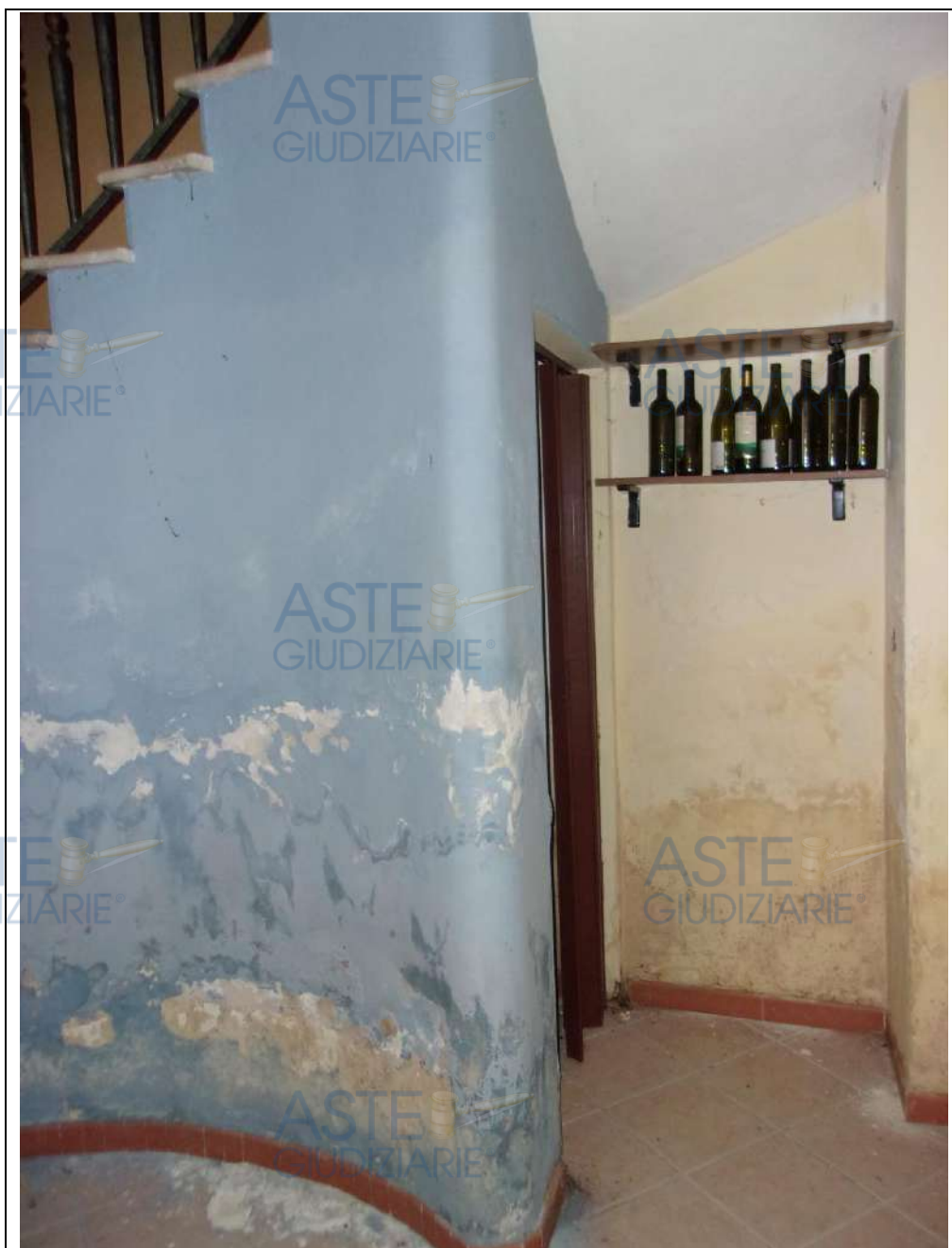
locale cisterna –piano terra
