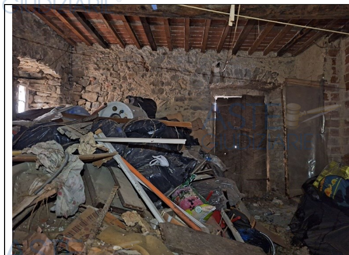
Cantina Piano terra
