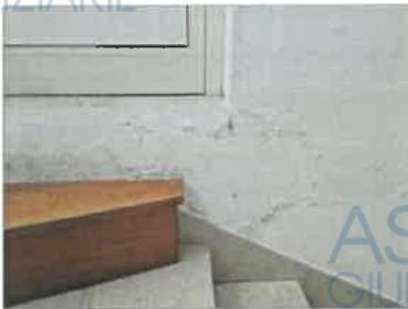
**FOTO 115** - UMIDITA' MURO SCALA
