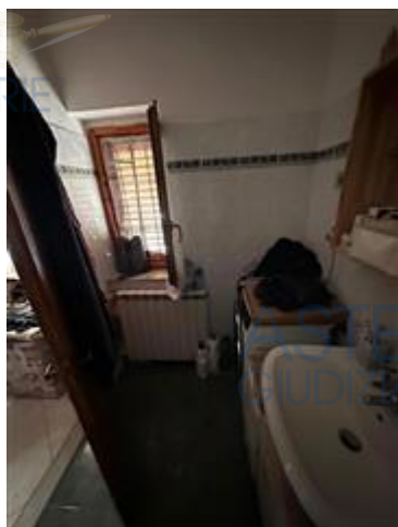
bagno piano terreno
